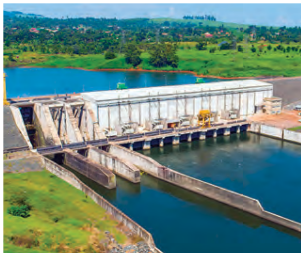
Bujagali run-of-river hydropower plant, Uganda
