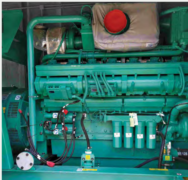
The gas engine of the recently installed Cummings C1400N6C generator at Savannah's Uquo CPF, Nigeria
