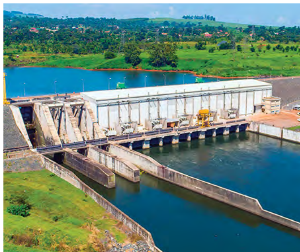
Bujagali run-of-river hydropower plant, Uganda
