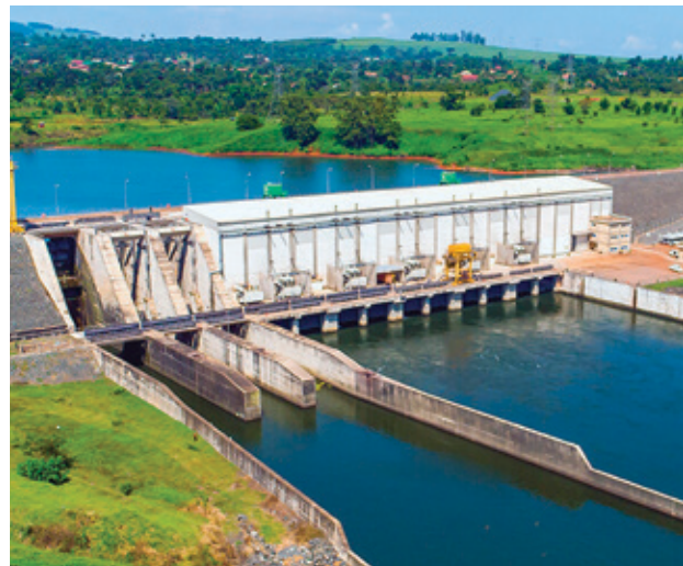
Bujagali run-of-river hydropower plant, Uganda
